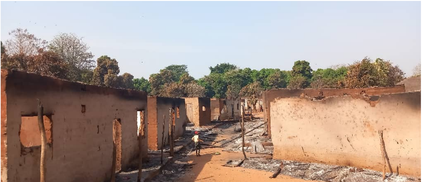
Image of burnt houses
